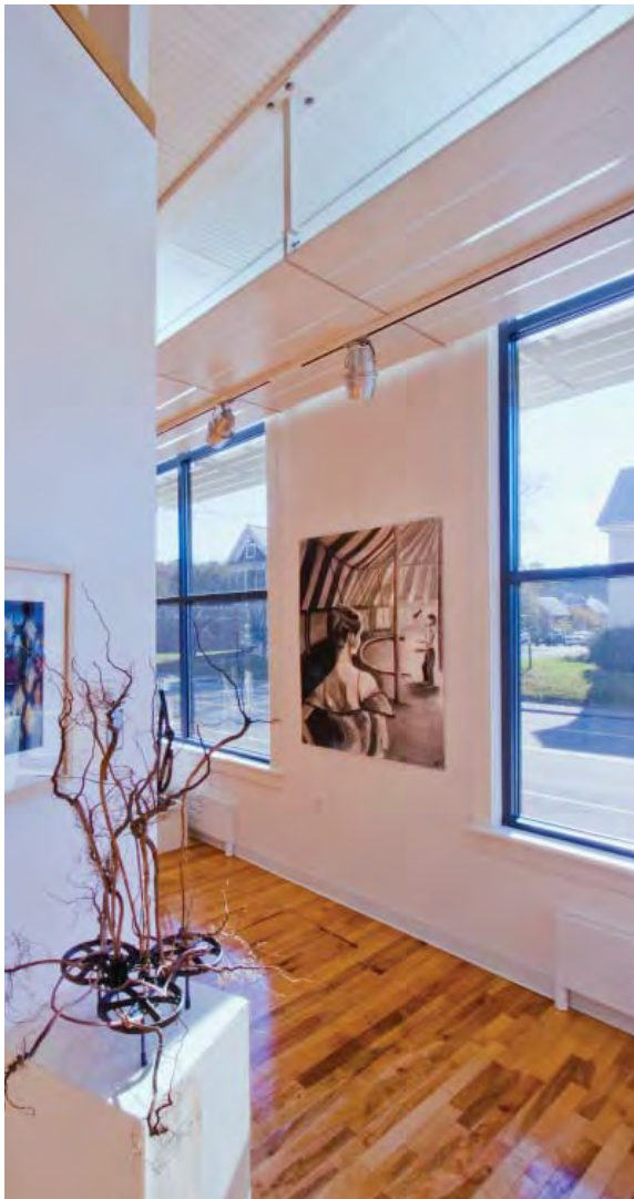
Interior Light Shelf - AVA Gallery and Art Center, LEED GOLD
