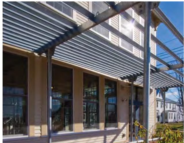
Exterior Sunshade- AVA Gallery and Art Center, LEED GOLD
